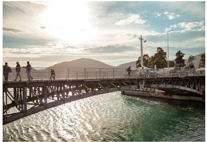
MOVING BRIDGE OF EURIPUS
